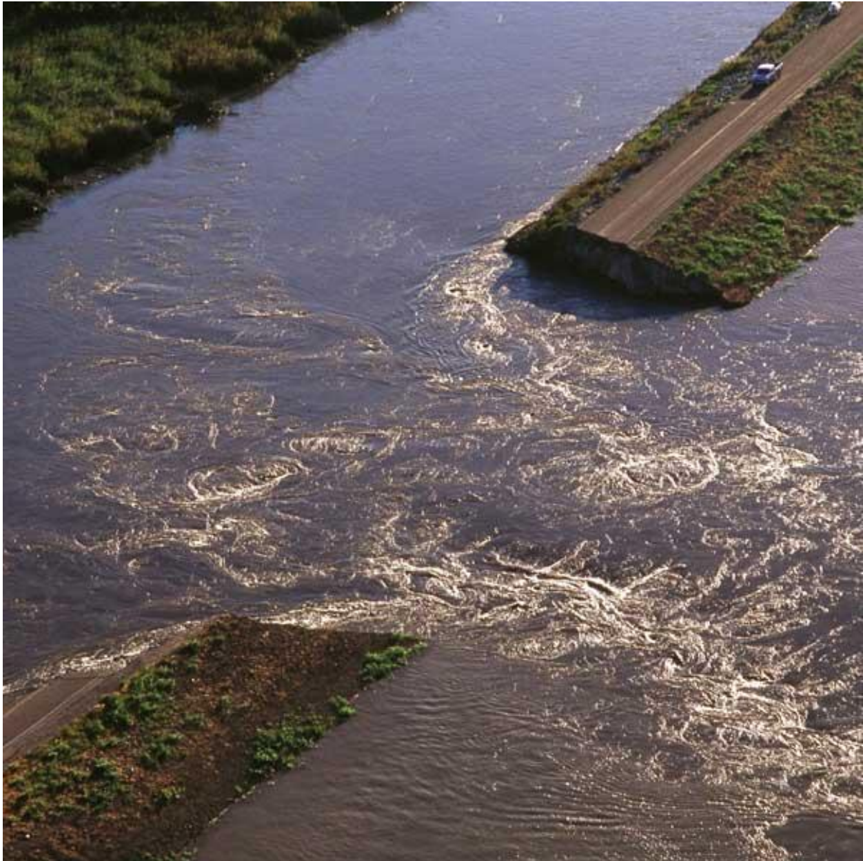
Figure 4.7. Levee Failure
